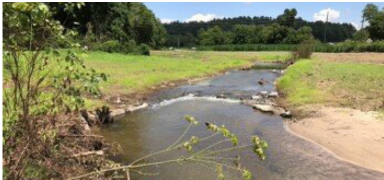
The Robinson Creek project employed several Natural Channel Design techniques. The project team realigned the channel and excavated the floodplain. They also installed log j-hook vanes, toe wood revetments, and cobble riffles.
