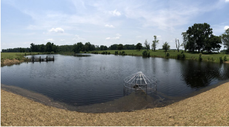
This agriculture pond sustained extensive damage from hurricanes in 2016. It was restored by Resource Institute under a program from the NC Department of Agriculture & Consumer Services.
