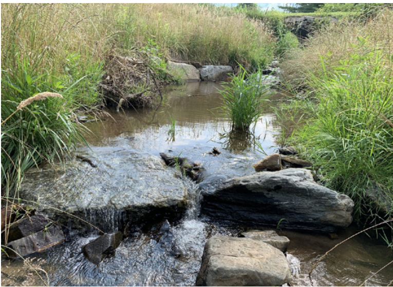
Instream structures constructed for the Linville Creek restoration project.
