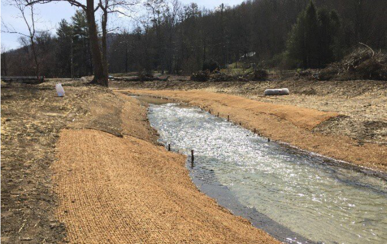
Shaw Creek in Henderson County, North Carolina after in-stream construction
