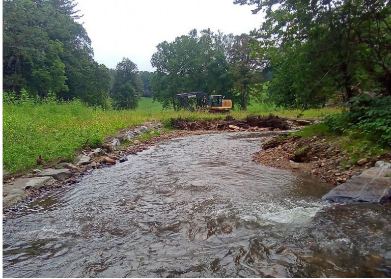
Little Crabtree Creek restoration during in-stream construction.
