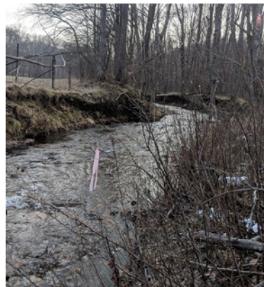
BEFORE: Streambanks on Call Creek were steep and severely eroded.
