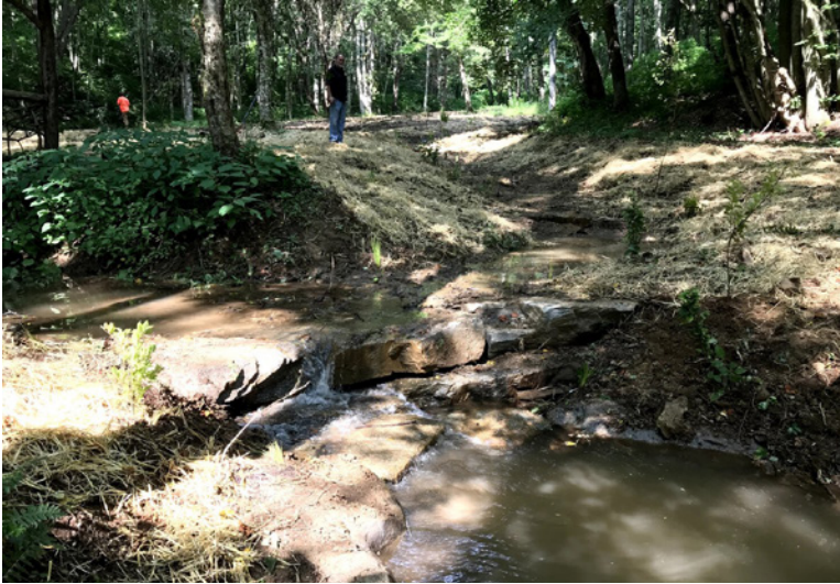
Instream structures constructed to stabilize Stingy Branch and create aquatic habitat.
