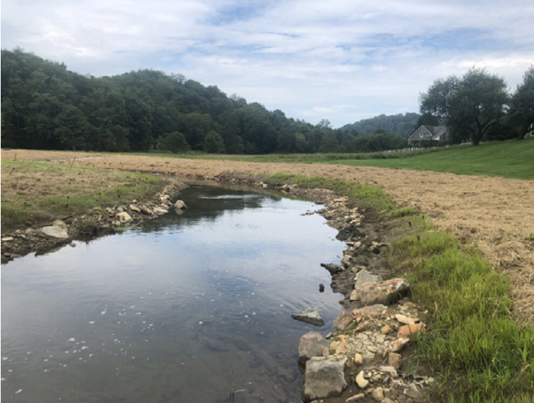
Resource Institute restored a reach of the Upper Elk River near Banner Elk, NC. The project is part of the North Carolina Stream Restoration Initiative.
