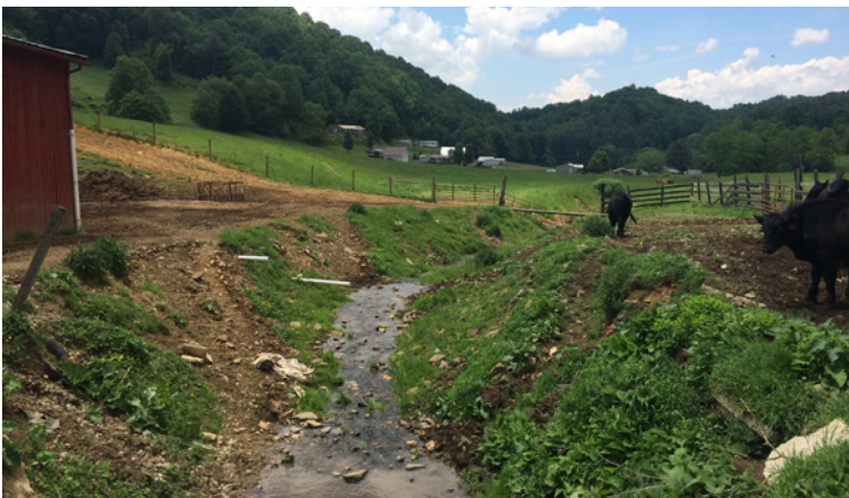
BEFORE: Linville Creek lacked stream crossings contributing to streambank and streambed erosion.
