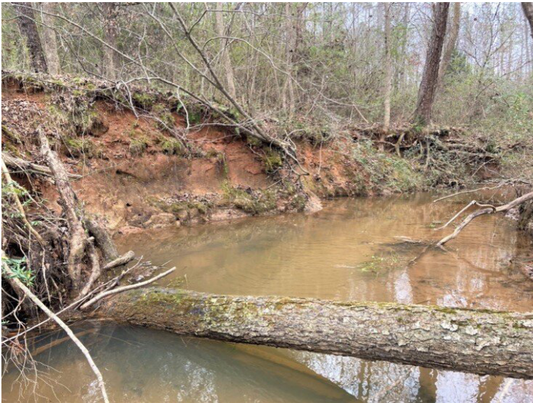
BEFORE: Prior to restoration, Leonard Creek's streambanks were steep and severely eroding and unstable.
