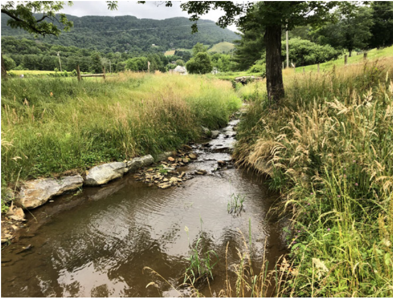
Linville Creek stream restoration project after instream construction and planting the riparian buffer.
