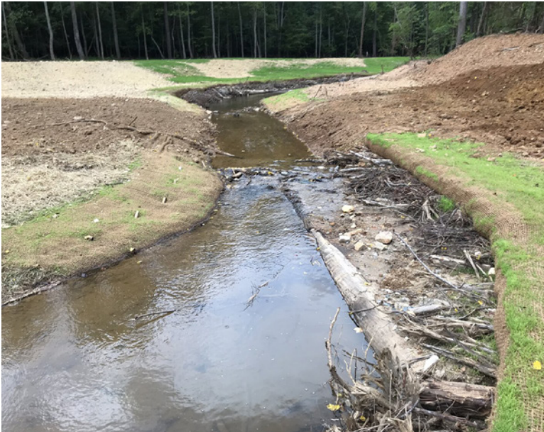
Instream structures constructed to stabilize Grassy Creek and create aquatic habitat.
