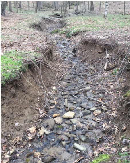
BEFORE: Prior to restoration Stingy Branch's streambanks were severely eroded and the stream unstable.
