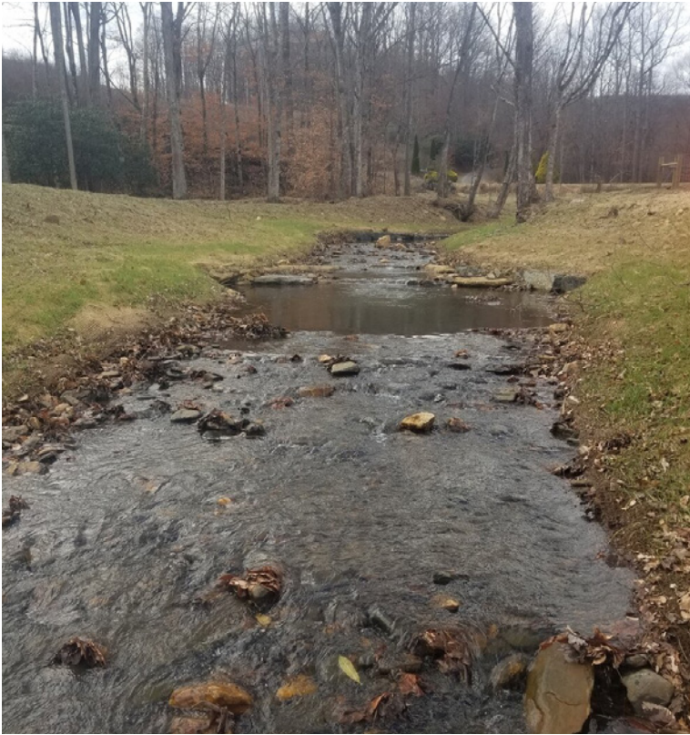
Call Creek post-restoration with stabilized streambanks and reconnected floodplain.
