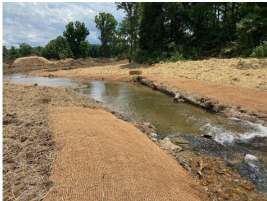
The Robinson Creek project employed several Natural Channel Design techniques. The project team realigned the channel and excavated the floodplain. They also installed log j-hook vanes, toe wood revetments, and cobble riffles.
