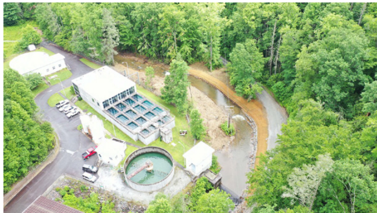
Aerial view of the Catheys Creek Project and the Brevard Water Treatment Plant. This view is after instream construction and prior to riparian planting.
