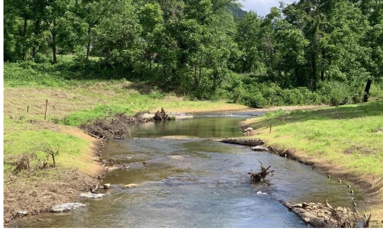
Reedy Patch Creek instream structures looking upstream, July 2020
