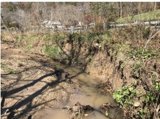
BEFORE: Originally, UT Foster Creek's severely eroding streambanks contributed to a high sediment load and poor water quality.
