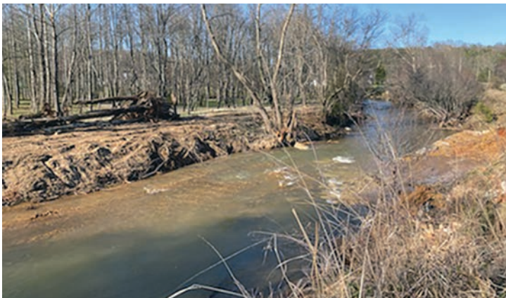
A reach of stream in Surry County, NC damaged by Hurricanes Florence and Michael in 2018. This photo was taken prior to the EWP recovery project.
