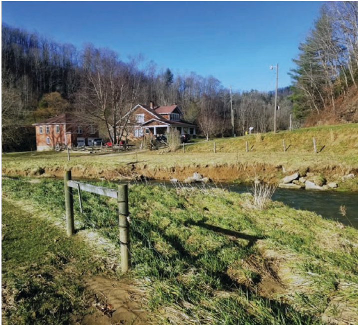
Cove Creek post-construction and prior to riparian buffer planting.
