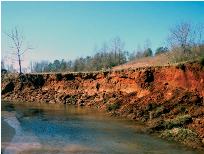
Prior to project implementation, Cleghorn Creek streambanks were steep and unstable.
