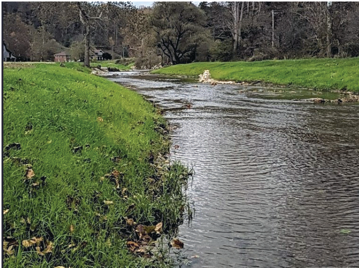
Prior to project implementation, Cove Creek streambanks were steep and unstable.
